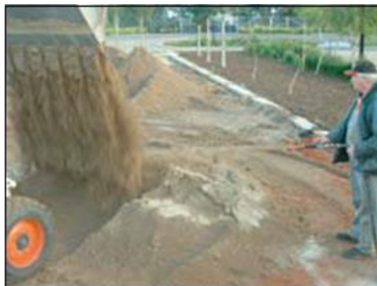
Mix Soilbond into granitic sand
