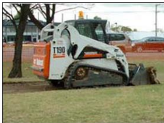
Excavate to required depth
