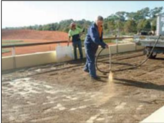
Side to side spraying using a hand lance ensuring coverage of the granitic sand path
