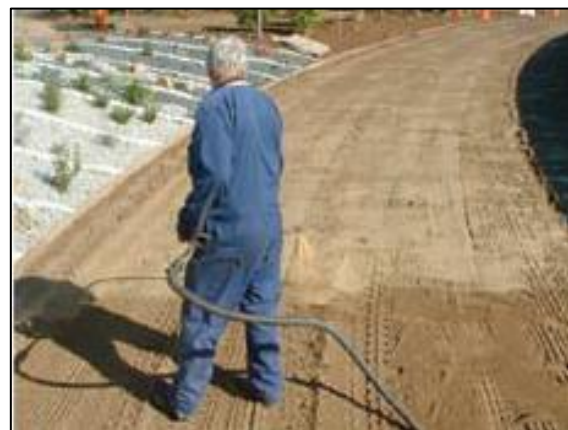
Even distribution of Soilbond A01 over the surface
