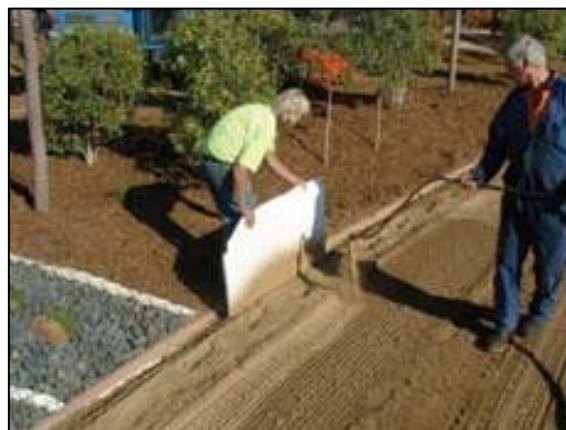
It is important that the edges are thoroughly coated with Soilbond A01
