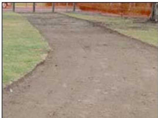
Surface ready for granitic sand
