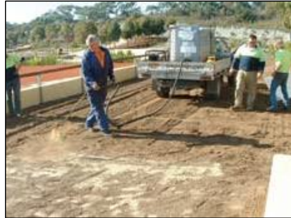
Side to side spraying using a hand lance ensuring coverage of the granitic sand path
